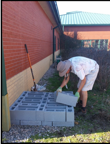
Step 1: Build a sturdy base to hold the water tank. This tank is 500 gallons. That's more than 4,200 lbs. of water!
